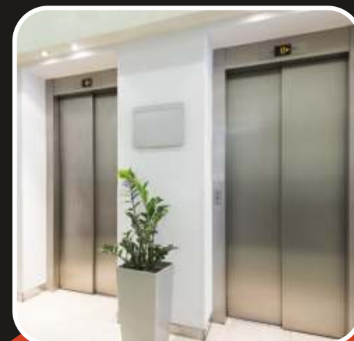
Lifts with power backup
