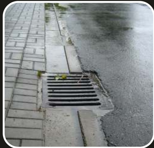
Storm water drainage
